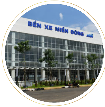
New Eastern Bus Station
